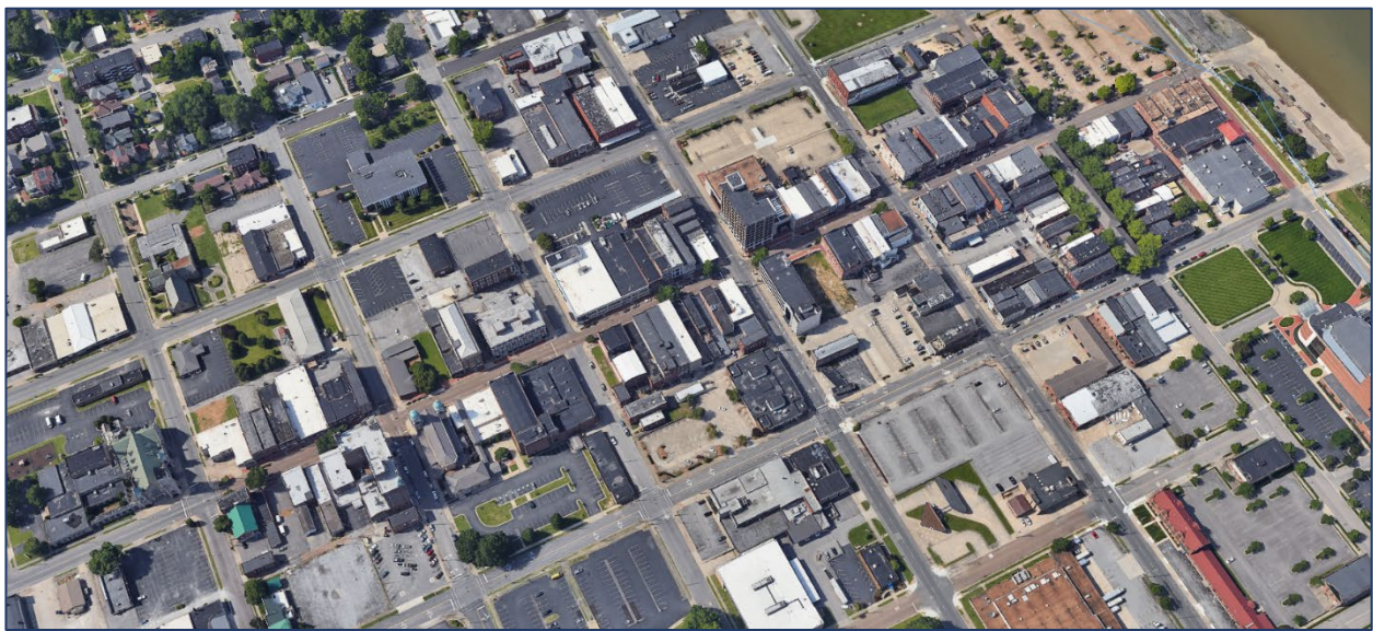
Classic Urban character focused along the Broadway Street corridor in Downtown Paducah, but quickly giving way to Auto Urban elements where surface parking takes up much or all of certain downtown blocks.
